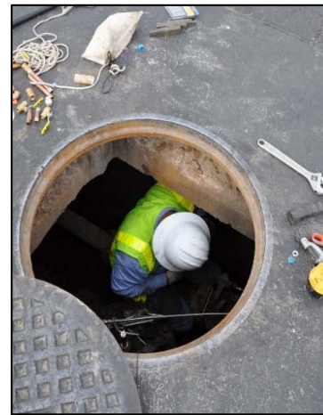
Image: Valve/Vault Repair
