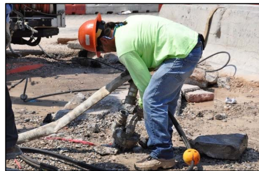
Image: LVVWD Field Repair
