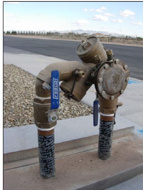
Image: Commercial Backflow Assembly
