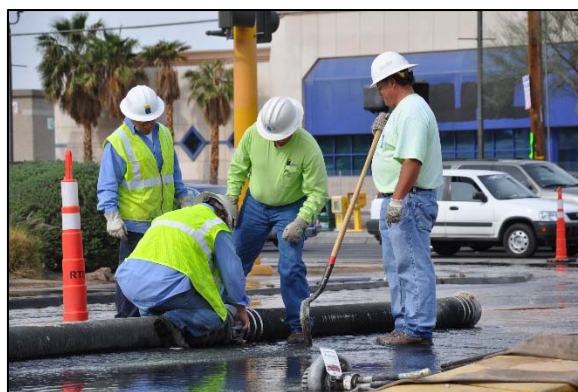
Image: LVVWD Pipeline Repair
