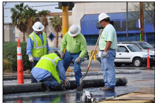
Image: LVVWD Pipeline Repair
