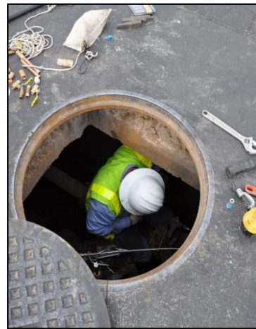
Image: Valve/Vault Repair
