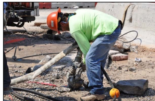
Image: LVVWD Field Repair
