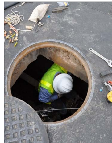
Image: Valve/Vault Repair
