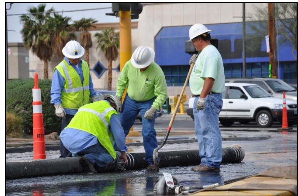
Image: LVVWD Pipeline Repair
