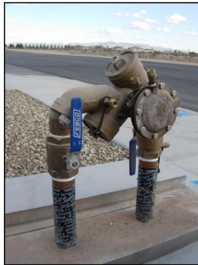
Image: Commercial Backflow Assembly
