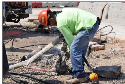
Image: LVVWD Field Repair
