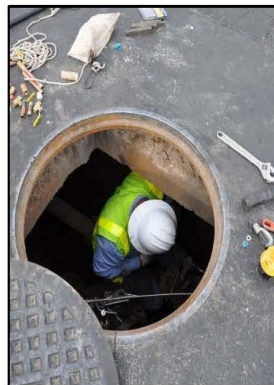
Image: Valve/Vault Repair
