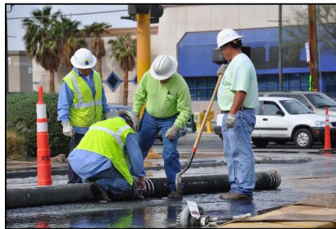
Image: LVVWD Pipeline Repair
