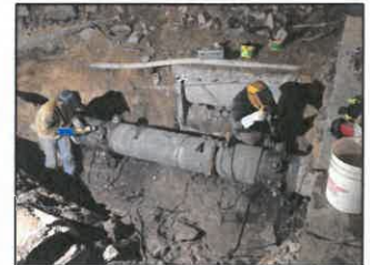
Crews address a main break on Las Vegas Boulevard
