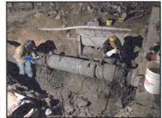
Crews address a main break on Las Vegas Boulevard
