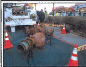
LVVWD crews performing meter replacements
