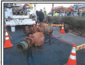
LVVWD crews performing meter replacements
