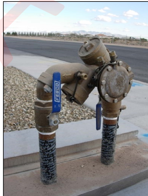
Image: Commercial Backflow Assembly
