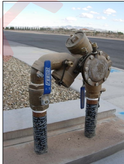
Image: Commercial Backflow Assembly
