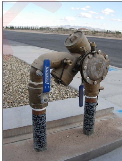
Image: Commercial Backflow Assembly
