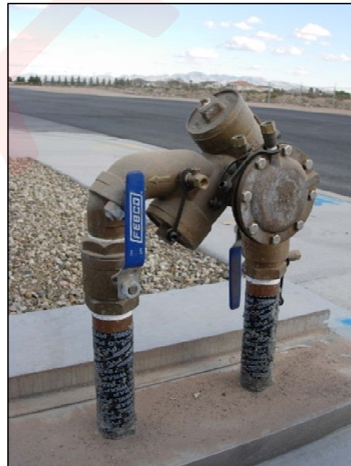
Image: Commercial Backflow Assembly
